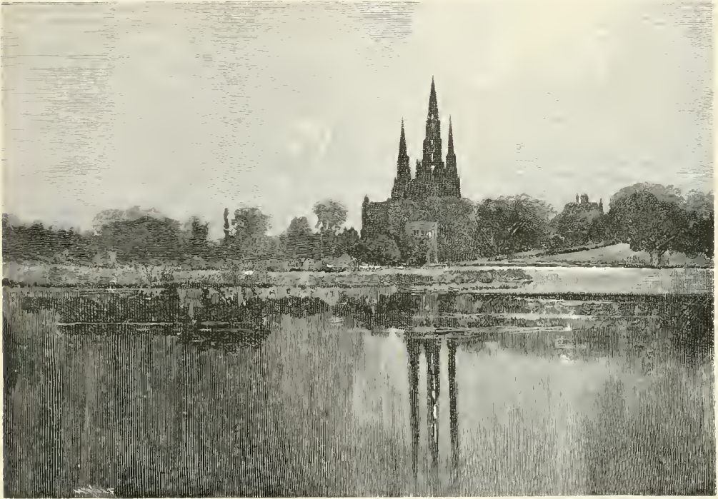
LICHFIELD CATHEDRAL, FROM THE EAST.
